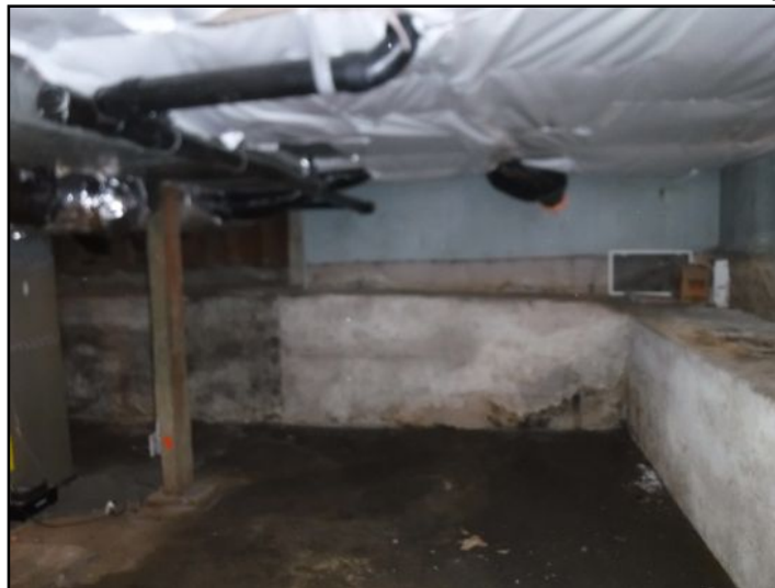
Basement foundation with slab floor and concrete perimeter walls
