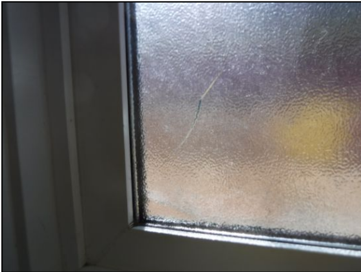
Single hung window in living room: Cracked glass noted. Recommend corrections to improve safety, security, access to light.
