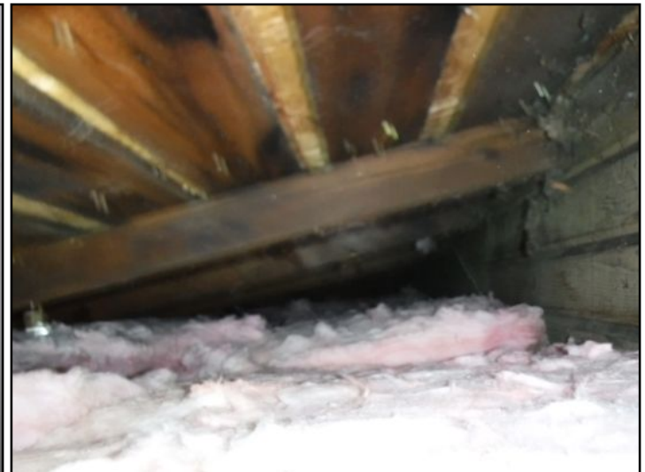
Access to attic was by Scuttle Hole located in: Laundry room
