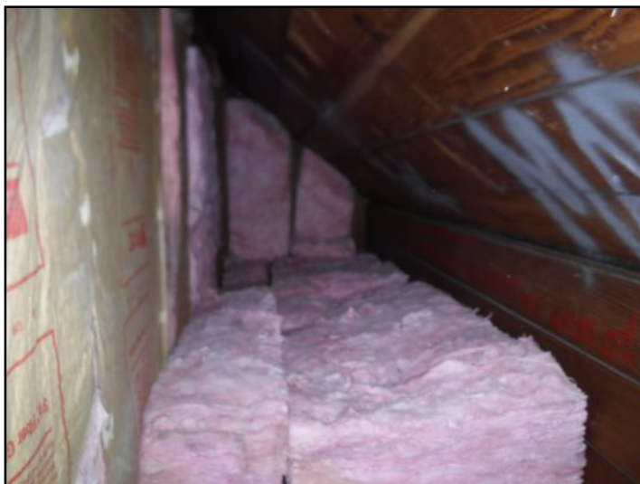
Access to attic was by Door or Hatch located in: Bedroom
